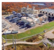
Towantic natural gas-fired thermal power plant
