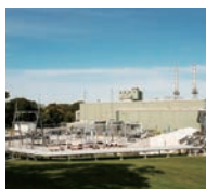
Michigan Power natural gas-fired thermal power plant
