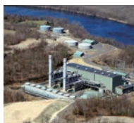
Kleen Energy natural gas-fired thermal power plant
