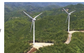
Inami Wind Power Plant
