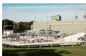
Michigan Power natural gas-fired thermal power plant
