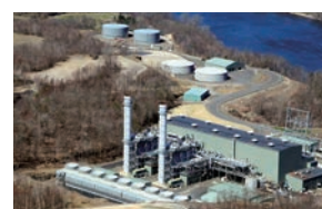
Kleen Energy natural gas-fired thermal power plant
