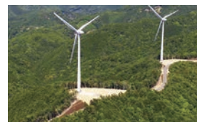
Inami Wind Power Plant
