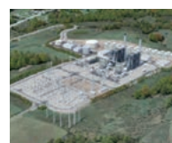
Fairview Power Plant
