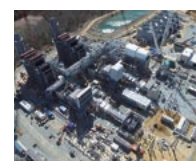
St. Charles Power Plant
