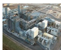
Shore Power Plant
