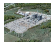
Fairview Power Plant
