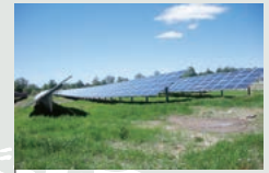
Aurora Solar Power Generation Project
