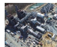
St. Charles Power Plant
