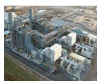
Shore Power Plant
