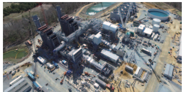
St. Charles Energy Center Natural Gas-Fired Power Plant (under construction)
