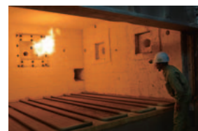
Experimental furnaces measure actual data
