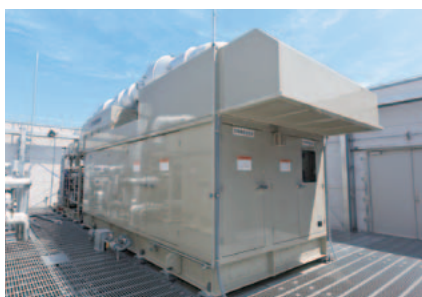
Gas cogeneration system
