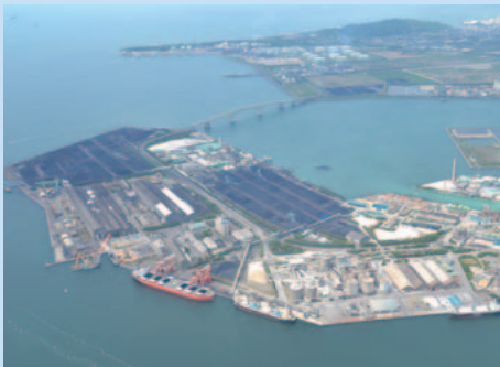
Yamaguchi-Ube Power Generation Generation capacity: 1.2 GW (planned) / Generation facilities: ultra supercritical pressure boiler (coal) / Start of operations: early 2020s (planned)
