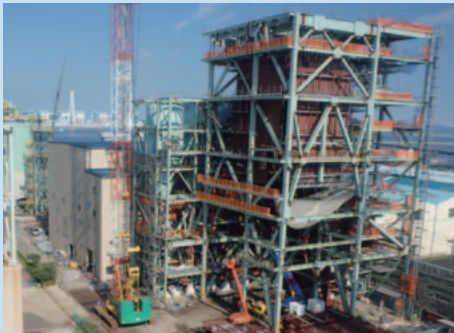
Nagoya II Power Plant (under construction), Nakayama Nagoya Joint Power Generation Generation capacity: 110 MW / Generation facilities: sub-critical pressure boiler (coal/wood biomass) / Start of operations: FY2017
