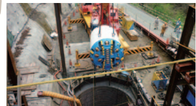
Pipeline open-cut construction work
