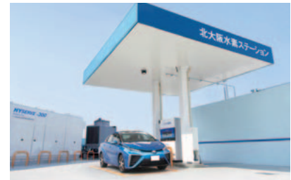
Kita-Osaka Hydrogen Station (Began operation in Ibaraki, Osaka in April 2015)
