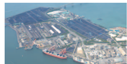
Yamaguchi Ube Power Coal-Fired Power Plant Generation capacity: 1.2 GW (planned) / Generation facilities: ultra supercritical pressure boiler / Start of operations: early 2020s
