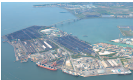
Yamaguchi Ube Power Coal-Fired Power Plant Generation capacity: 1.2 GW (planned) / Generation facilities: ultra supercritical pressure boiler / Start of operations: early 2020s
