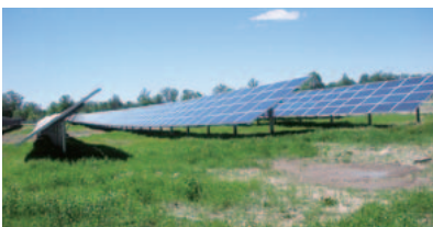
Aurora Solar Power Plant (Canada)
