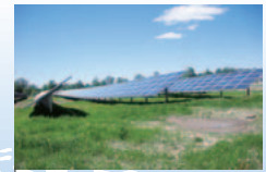
Aurora Solar Power Generation Project
