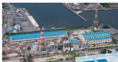
Expansion of Nakayama Nagoya Joint Power Generation Coal-Fired Power Plant Operation at 110 MW to begin in 2016
