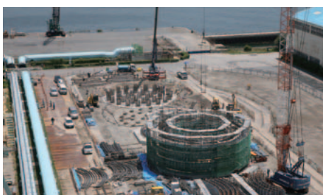
Expansion of Nakayama Nagoya Joint Power Generation Coal-Fired Power Plant (under construction) Generation capacity: 110 MW / Generation facilities: sub-critical pressure boiler (biomass multi-fuel combustion) / Start of operations: Second half of FY2016
