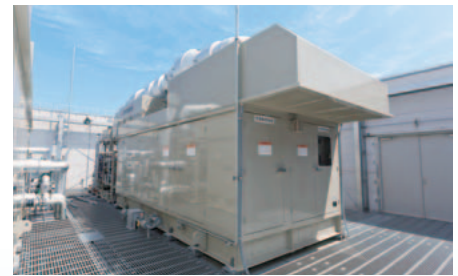
Gas cogeneration system
