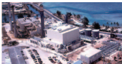
Marianas Energy Power Plant (USA)
