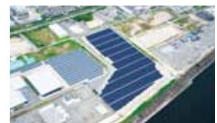
Torishima Solar Power Plant
