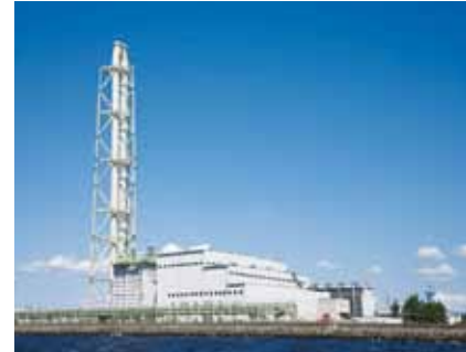
Senboku Natural Gas Power Plant
