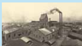
Foundation / commenced gas operations
