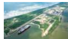
Photograph courtesy of Freeport LNG Development, L.P
