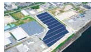
Torishima Solar Power Plant
